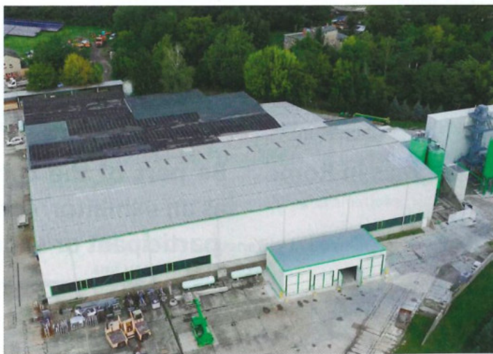
Fig. 1: A bird's-eye view of the Mattig & Lindner precast concrete plant in Forst/Lusatia
