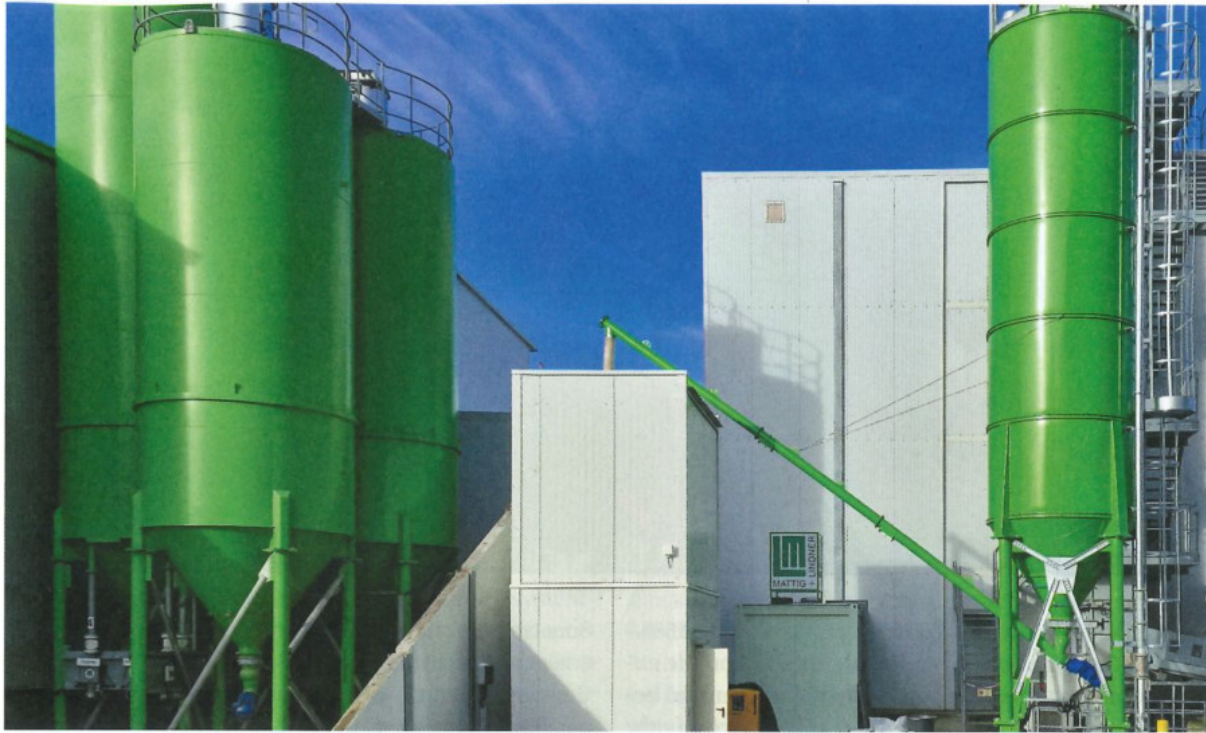
Fig. 2: Extensive modernization measures were recently carried out
